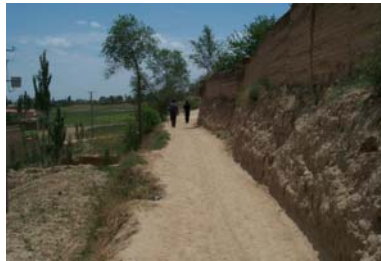
This path with a steep 8-12 foot drop-off goes in to the mid-level of He Jia Gou Village, which is accessible on foot, by bicycle, or by motorcycle.
