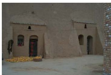
The front wall forming the entrance to their hand-hewn cave-like rooms
