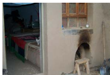
A special brick bed with a fire underneath keeps the family warm in the winter
